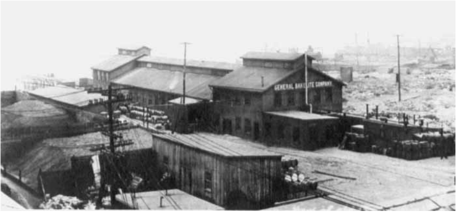
FIG. 10. General Bakelite Company's 1911 expanded facilities in Perth Amboy, New Jersey.
